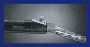
The strap of the cable sheath is insulated beyond the strap end by means of an insulation strip of approx. 10mm. The covering plate must be fixed with the wide side towards the sheath opening by means of a self-locking nut, ensuring simultaneously the attachment of the base and the contact plate in the cable.
