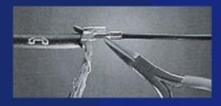
The shield connection clip is placed on the cable sheath between the cores and the inside of the cable sheath by means of a pair of tongs.
